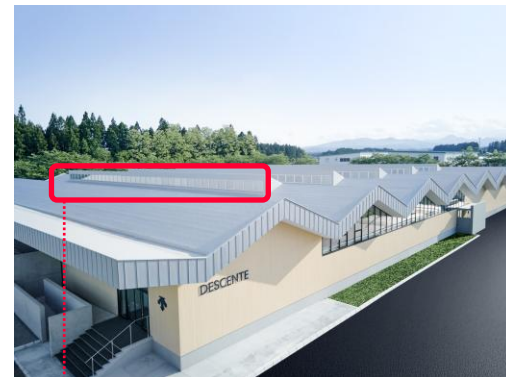
“Light-Diffusion Films” adopted for skylights at the Mizusawa Plant of Descente Apparel
