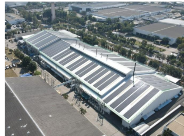
Solar panels installed at a plant in Thailand (ECT)
